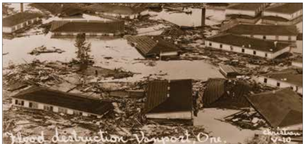
Flooded apartments during the Vanport Flood of 1948. (Photo courtesy of Oregon Historical Society)
