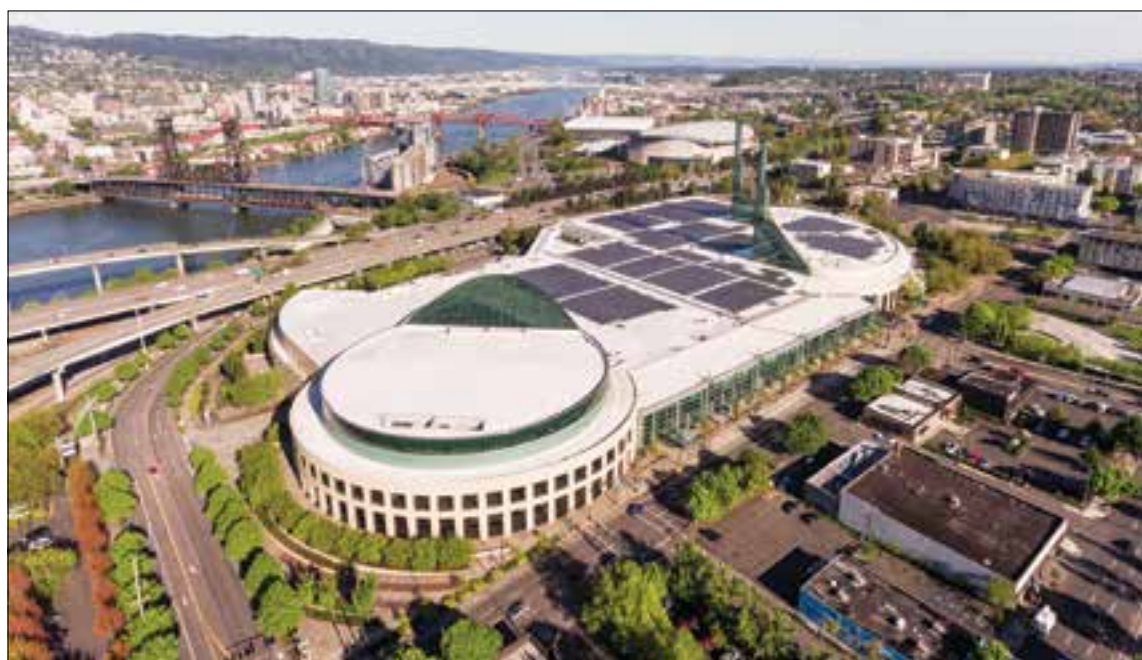
The Oregon Convention Center in northeast Portland.
