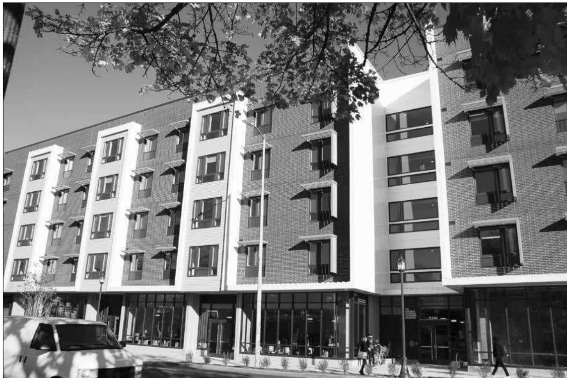
The new Beatrice Morrow apartment building at 3368 N.E. Martin Luther King Jr. Blvd. is housing developed by the African-American led non-profit, Portland Community Reinvestment Initiatives, Inc. (PCRI) and its pathway 1000 initiative, a 10-year plan to construct 1,000 new affordable homes and rentals, in particular for minority residents who have been displaced from inner north and northeast Portland.
