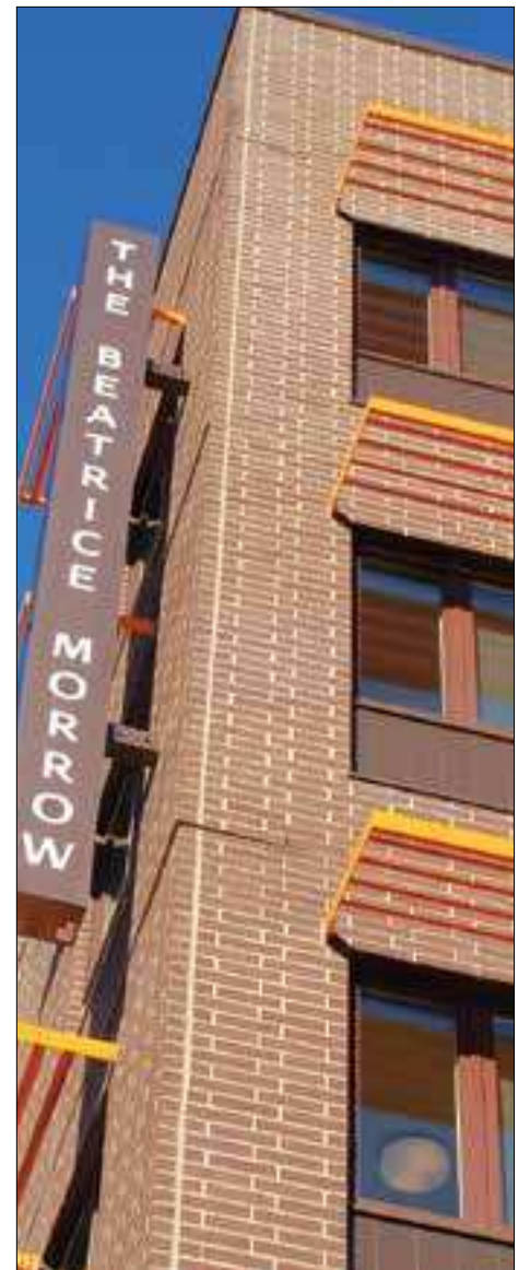
The Beatrice Morrow's affordable apartments at Northeast Martin Luther King Jr. Boulevard and Cook Street are the first to open under the city's new right-to-return policy for displaced African American residents.
