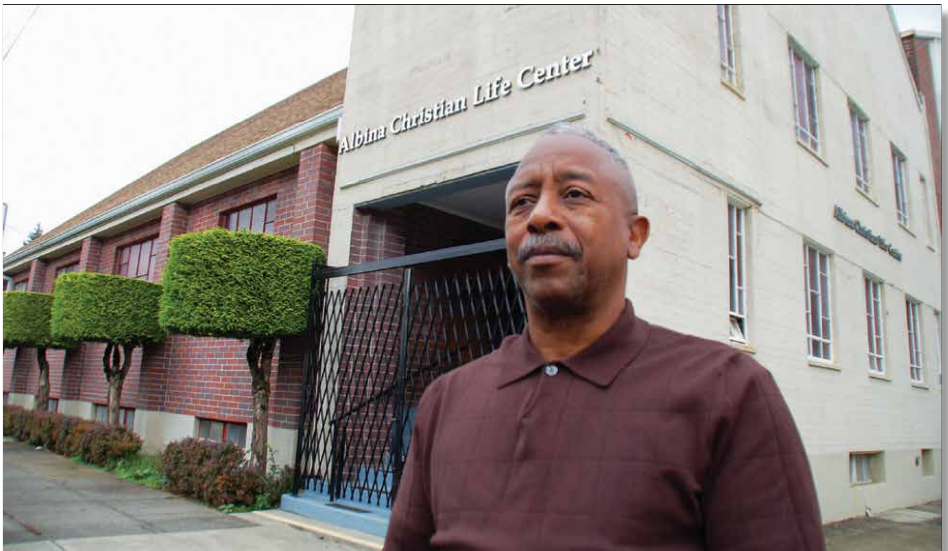
The Albina Christian Life Center in north Portland is one of a number of historically black churches in Portland that do not meet new earthquake safety standards, along with hundreds of other commercial buildings and several schools. Bishop Marcus Irving, pastor of the Albina center, says the cost to make $1 to $1.75 million in upgrades to the church would be difficult to obtain and fears that could trigger the city to condemn the church building or force it to close.
