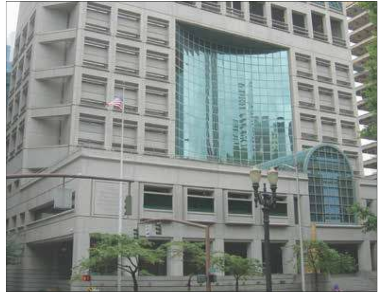
The Multnomah County Justice Center, downtown, includes a jail with several floors reserved for prisoners.
