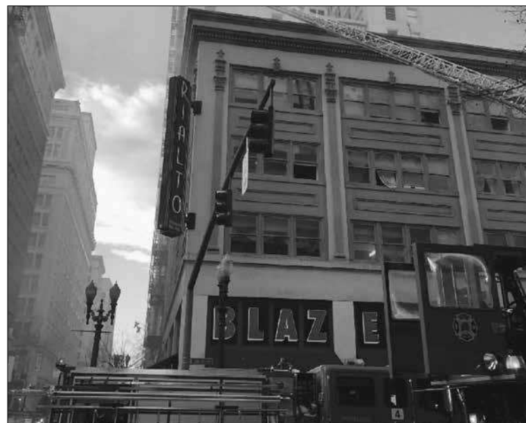
Firefighters respond when a fire erupts at the Hotel Alder, displacing low-income housing residents, downtown.
