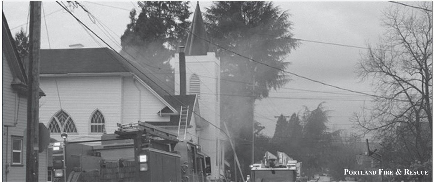
Firefighters did what they could to quell the fire that devastated the Allen Temple C.M.E. Church in February of last year.
