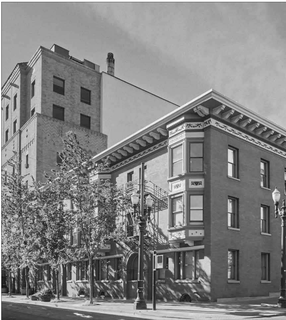
The 50-unit Bronaugh Apartments, downtown, celebrates a grand reopening as a home to elderly and disabled residents living on fixed incomes.
