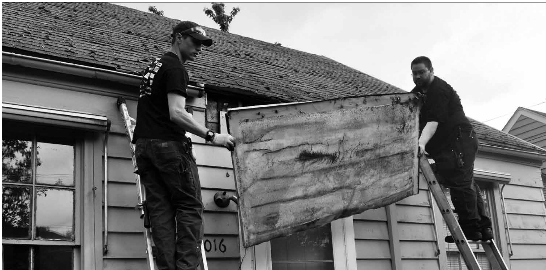
Kris Andrzejewski (left) and Toby Service remove a front door awning that was leaking and causing dry rot as part of a volunteer crew working to make repairs to the north-east Portland home of a low-income and disabled woman.
