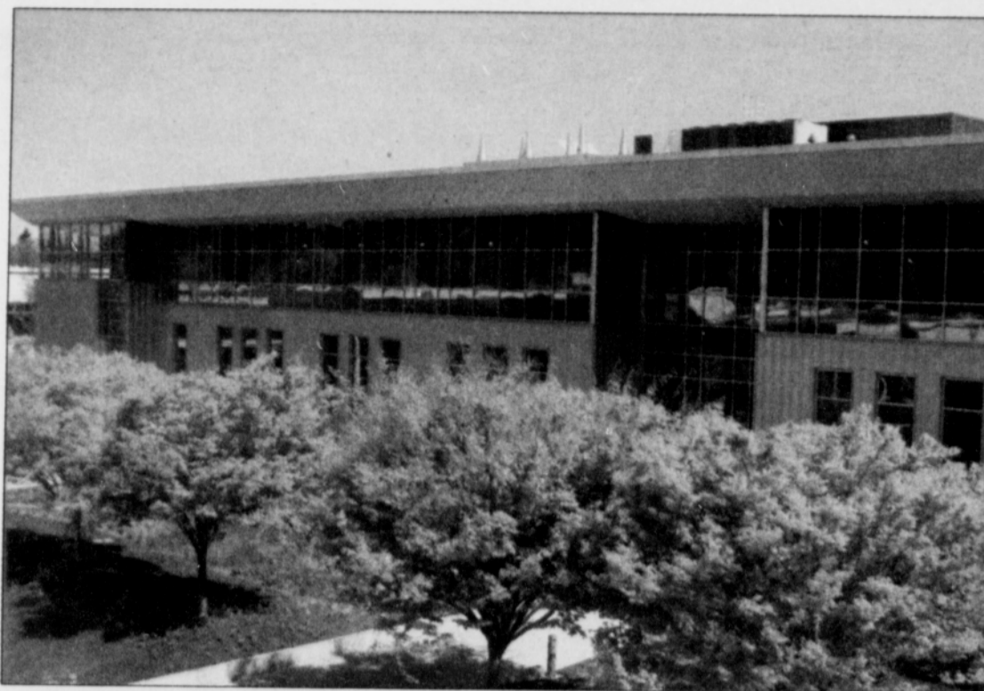
The new Portland Community College Student Commons on its southeast Portland campus is a three-story, 66,000-square-foot structure finished last spring that houses an expanded bookstore, five science classrooms with labs, six general purpose classrooms, four career technical education and computer classrooms and a new STEM (science, technology, engineering, and mathematics) Center.
