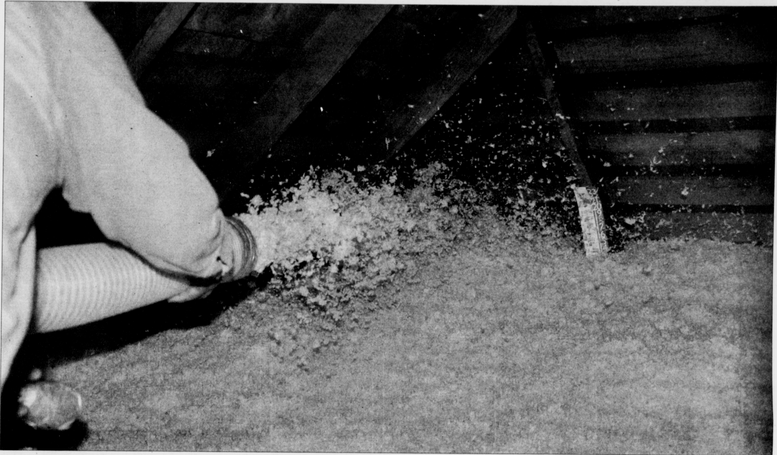
The non-profit Community Energy Project is offering Do-It-Yourself weatherization workshops for energy saving tasks such as blowing insulation into attic.
