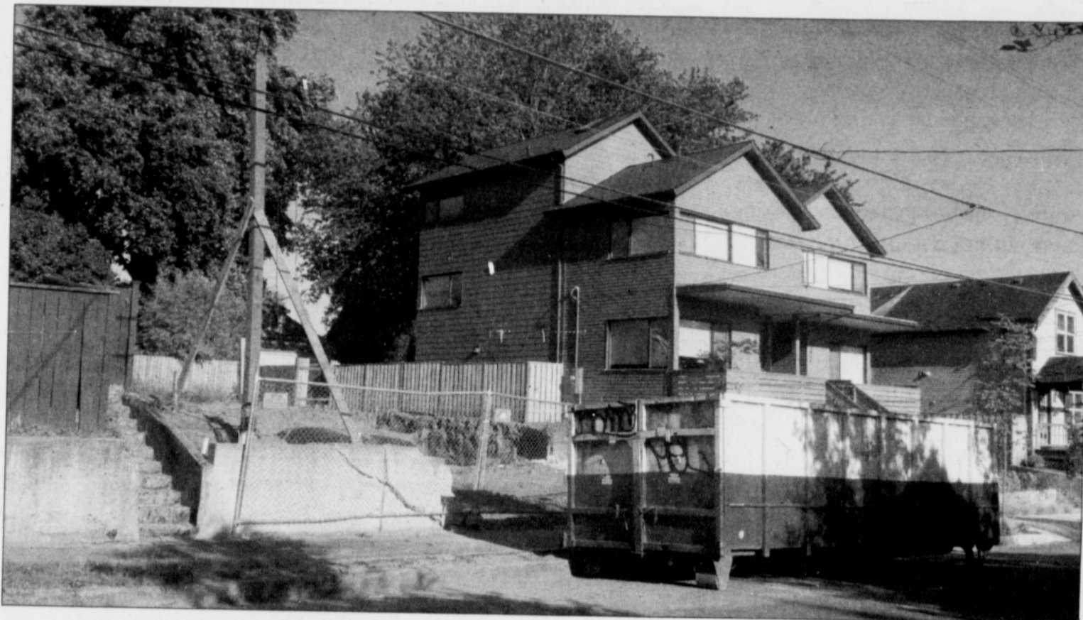
PHOTO BY COLIN STAUB/THE PORTLAND OBSERVER A demolished lot sits where a home stood to make way for new and more expensive housing near Northeast Eighth Avenue and Failing Street. The same thing happened next door (right), where two new rowhouses were built and sold in 2013 for $522,000 and $536,326, respectively.
