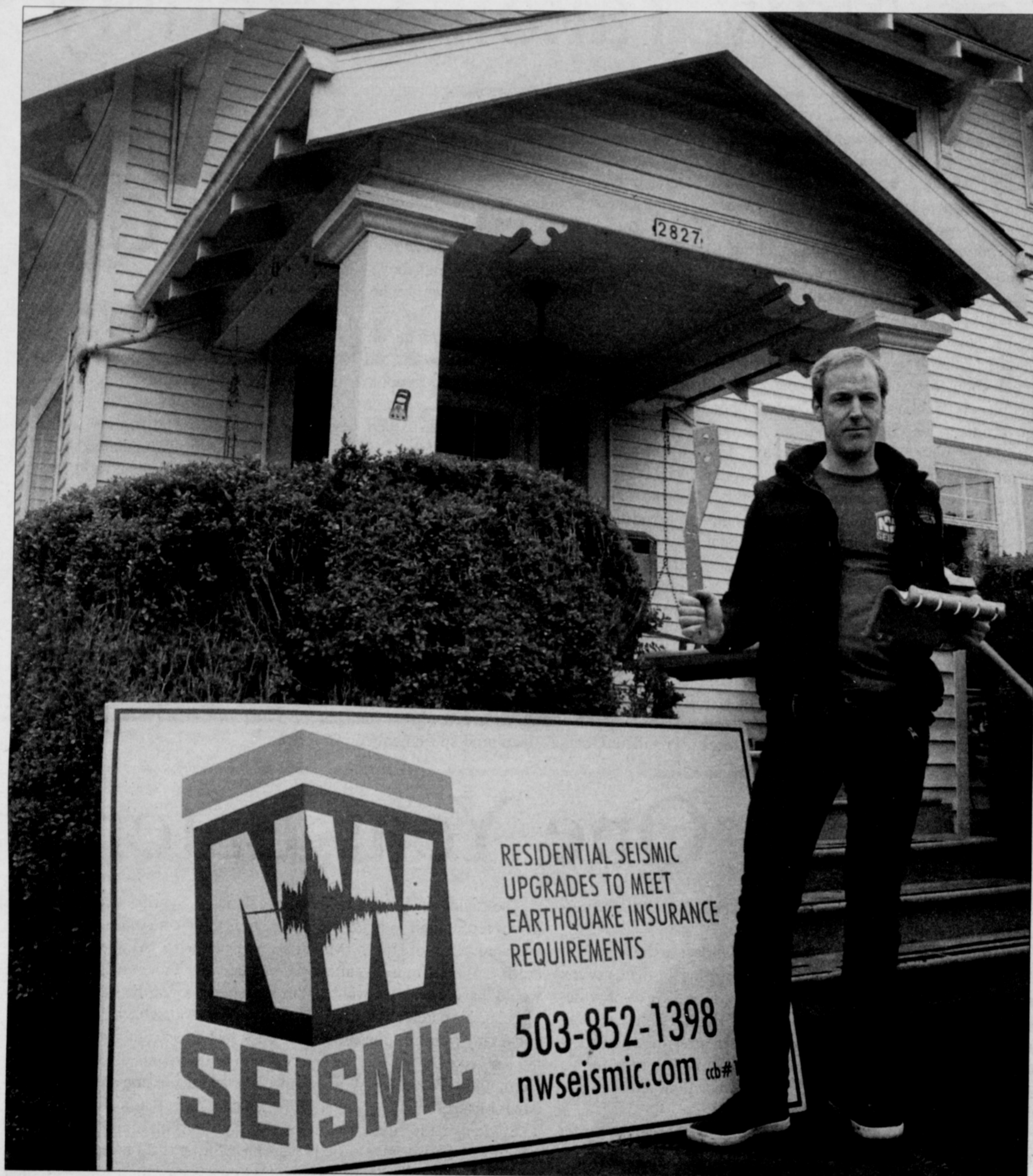
PHOTO BY CARI HACHMANN/THE PORTLAND OBSERVER Michael Wieber, owner of NW Seismic, shows what works and what doesn't when it comes to seismically retrofitting homes to withstand damages from a major earthquake, such as bolting a home to its foundation to resist lateral shifting.
