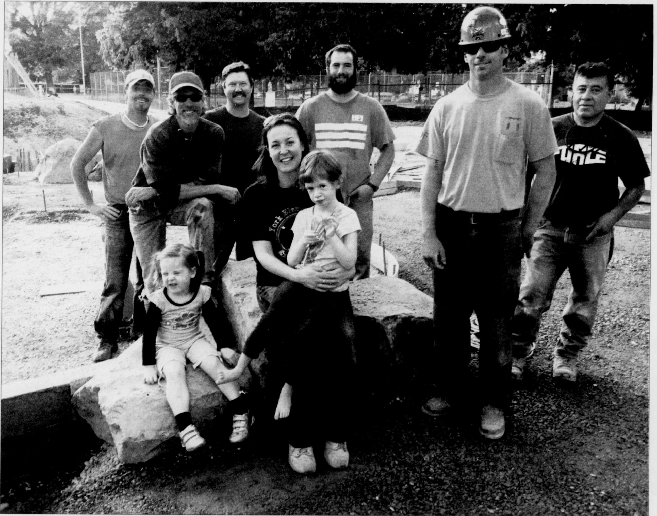
Harper Goldberg (center), her mother April Goldberg (seated), and her sister Lennon (left), join the construction crew during the installation of an all-inclusive play structure featuring wheelchair and walker-friendly elements at Arbor Lodge Park at North Bryant Street and Delaware Avenue.
