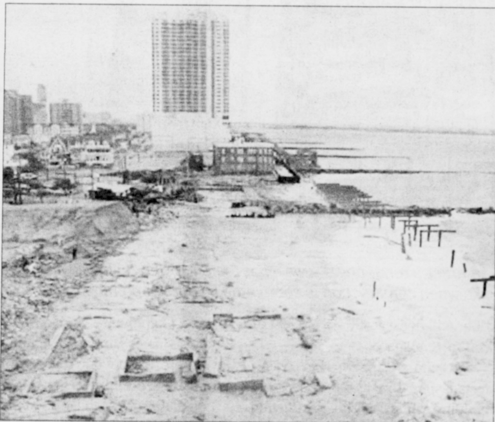
Foundations and pilings are all that remain of brick buildings and a boardwalk in Atlantic City, N.J., after they were destroyed when a powerful storm that started out as Hurricane Sandy made landfall on the East Coast on Monday night.
