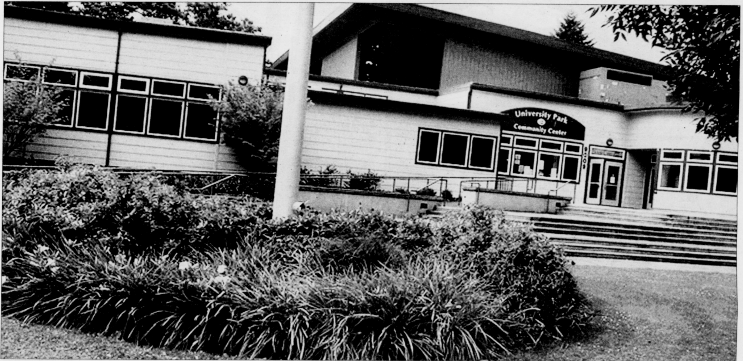
The University Park Community Center in north Portland will be renamed in honor of Charles Jordan, the former Portland City Commissioner and Director of Portland Parks and Recreation. Jordan has been a champion for children, families and building community.
