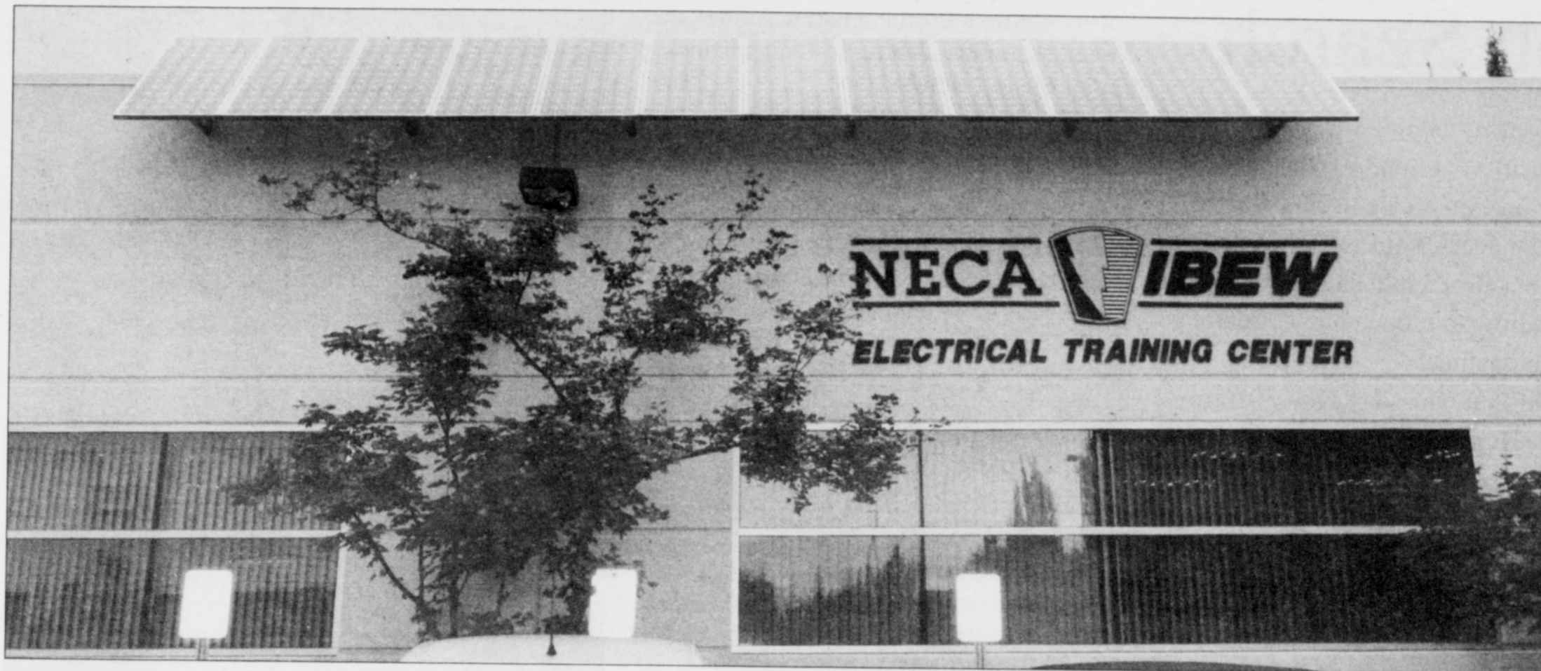
The NECA/IBEW Electrical Training Center with its new solar panel.
