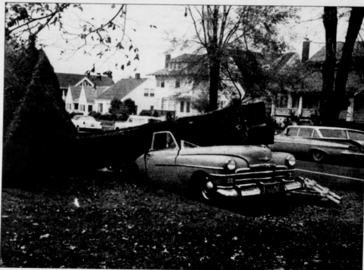
A photo from the city of Portland's Auditor's office shows damage from the 1962 Columbus Day Storm.
