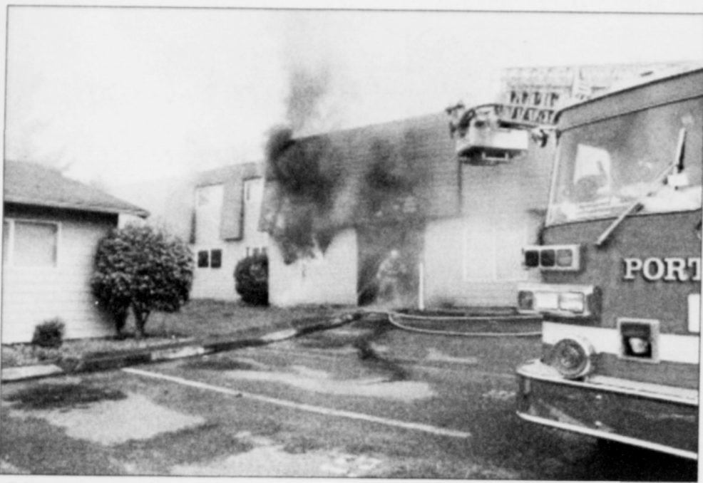
Officials said a pan left on the stove of a downstairs unit caused a fire that killed a woman in an upstairs unit at the Normandy Apartments at Northeast 46th and Killingsworth.
