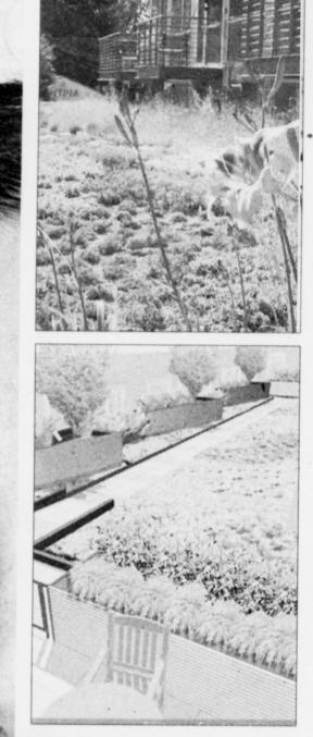
Two examples of an ecoroof. An ecoroof is a lightweight, low-maintenance, vegetated roof that provides stormwater management by capturing, filtering and evaporating rainfall.
