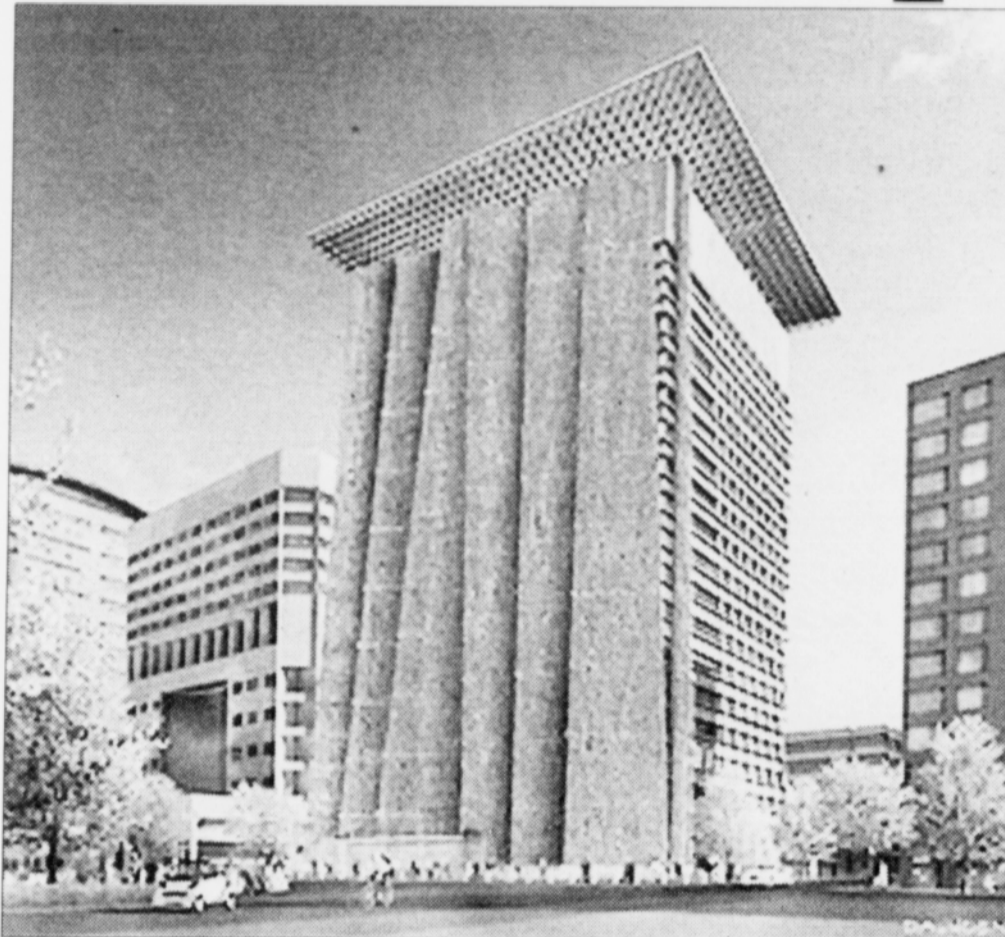
A computer generated image shows a series of 250-foot-tall trellises designed to shade the west side of the 18-story Edith Green-Wendell Wyatt Federal Building, downtown.
