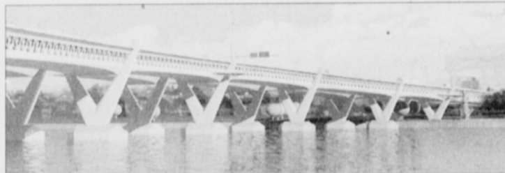
An artist's rendering shows the design concept for a new I-5 bridge over the Columbia River. Highway traffic would go on the top span with a path for walkers and bikes on the lower span.
