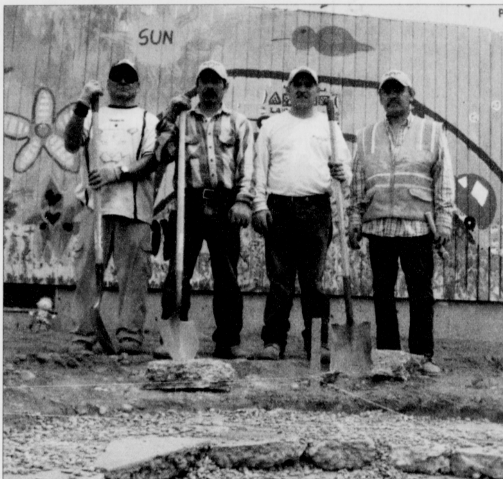
Workers stand near a bioswale, a form of "green" environmental construction meant to catch polluted rain water outside of Rigler Elementary School in northeast Portland. The men are in a program offered by Verde, a non-profit that offers green landscape training to traditionally marginalized groups.
