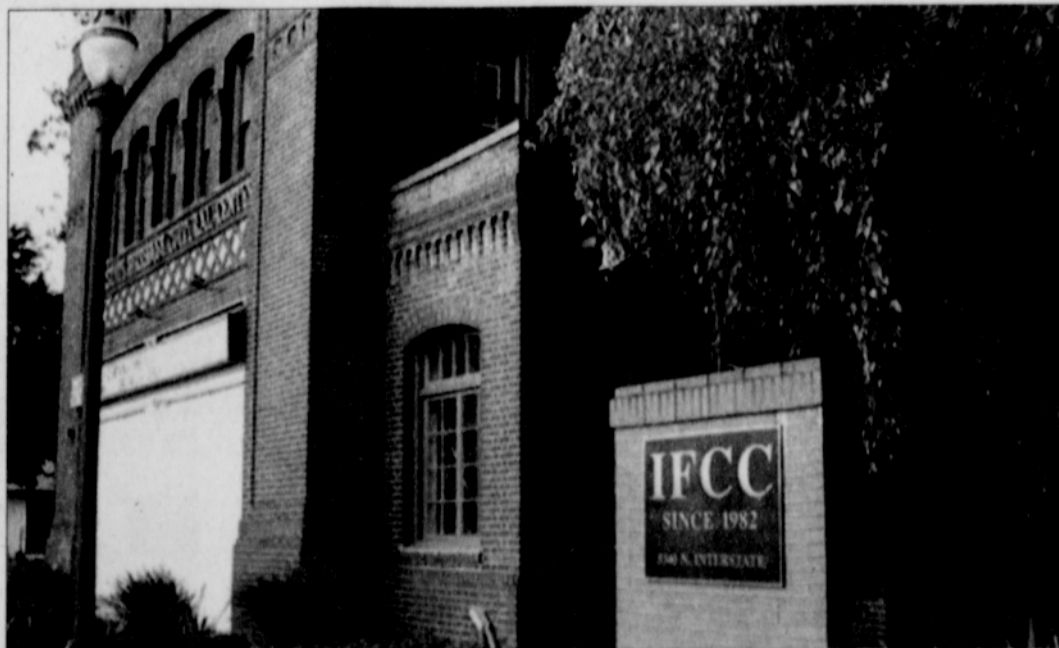
The Interstate Firehouse Cultural Center in north Portland is celebrating its 25th anniversary.
