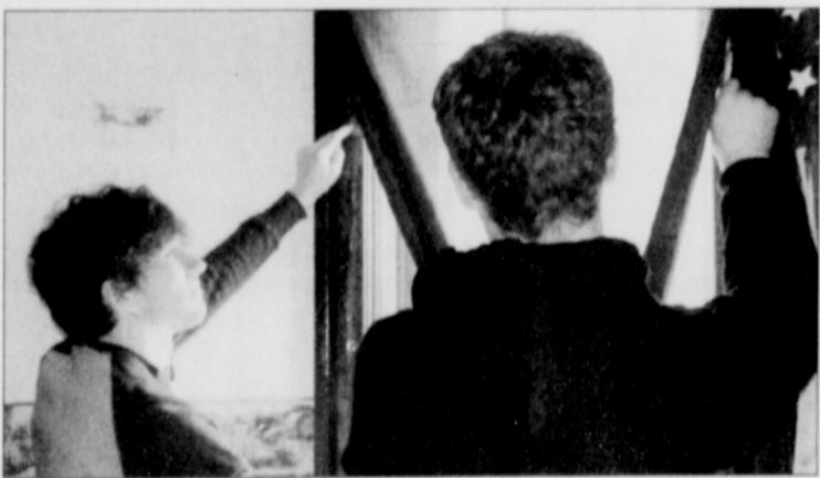
Plastic sheeting helps keep the heat in during winter and the air cool in the summer.
