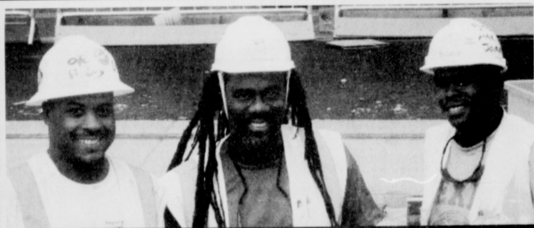
Jean Malary, owner of Affordable Electric, and crew provides duct bank work.
