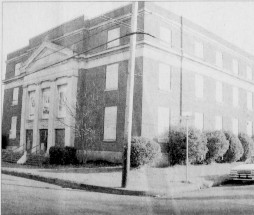
The dilapidated Masonic Temple on North Commercial Avenue across from Jefferson High School has been purchased by McMenamins. The local brew pub empire just opened its latest restaurant and bar next door to the site at the former Killingsworth Chapel of the Chimes.
