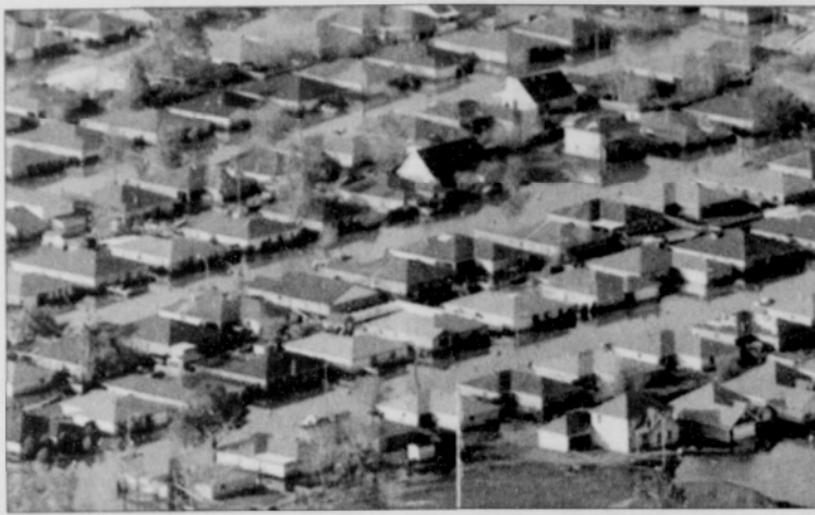
Neighborhoods are flooded with oil and water two weeks after Hurricane Katrina went through New Orleans. (AP photo)
