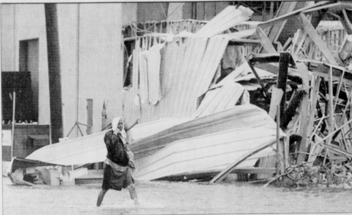
James Smith wades past a storm damaged building in Gulfport, Miss. After Hurricane Katrina.
