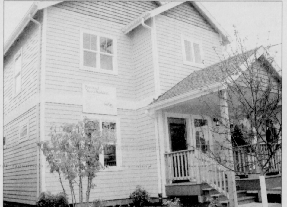
A partnership between advocates of vocational training for youth and affordable housing for adults resulted in the construction of this new at Northeast Sixth Avenue and Killingsworth Court.
