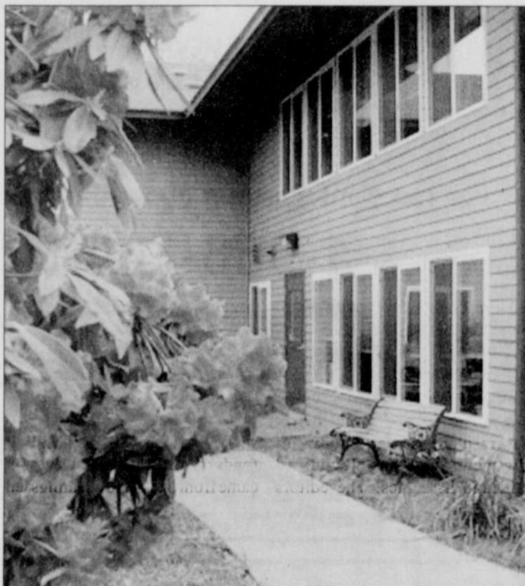
Prescott Terrace opens this month in northeast Portland, offering 48 units of housing as part of a 10-year plan to end homelessness.
