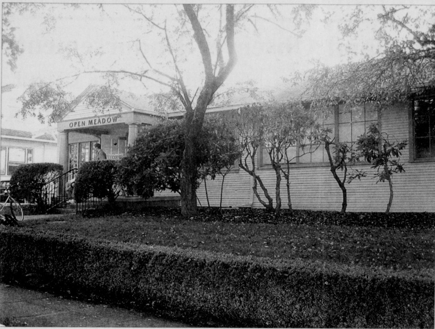
A newly renovated building serves Open Meadow, an alternative school in north Portland.
