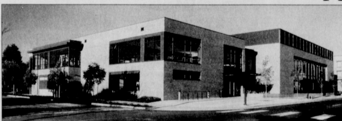
A new gym and physical education building is one of three new or remodeled structures to serve students this fall on the PCC Cascade campus at 705 N. Killingsworth St.
