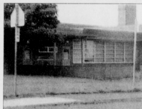
New shops and other upgrades will make Meek Elementary on Northeast Alberta Court a high school for Vocational Village.
