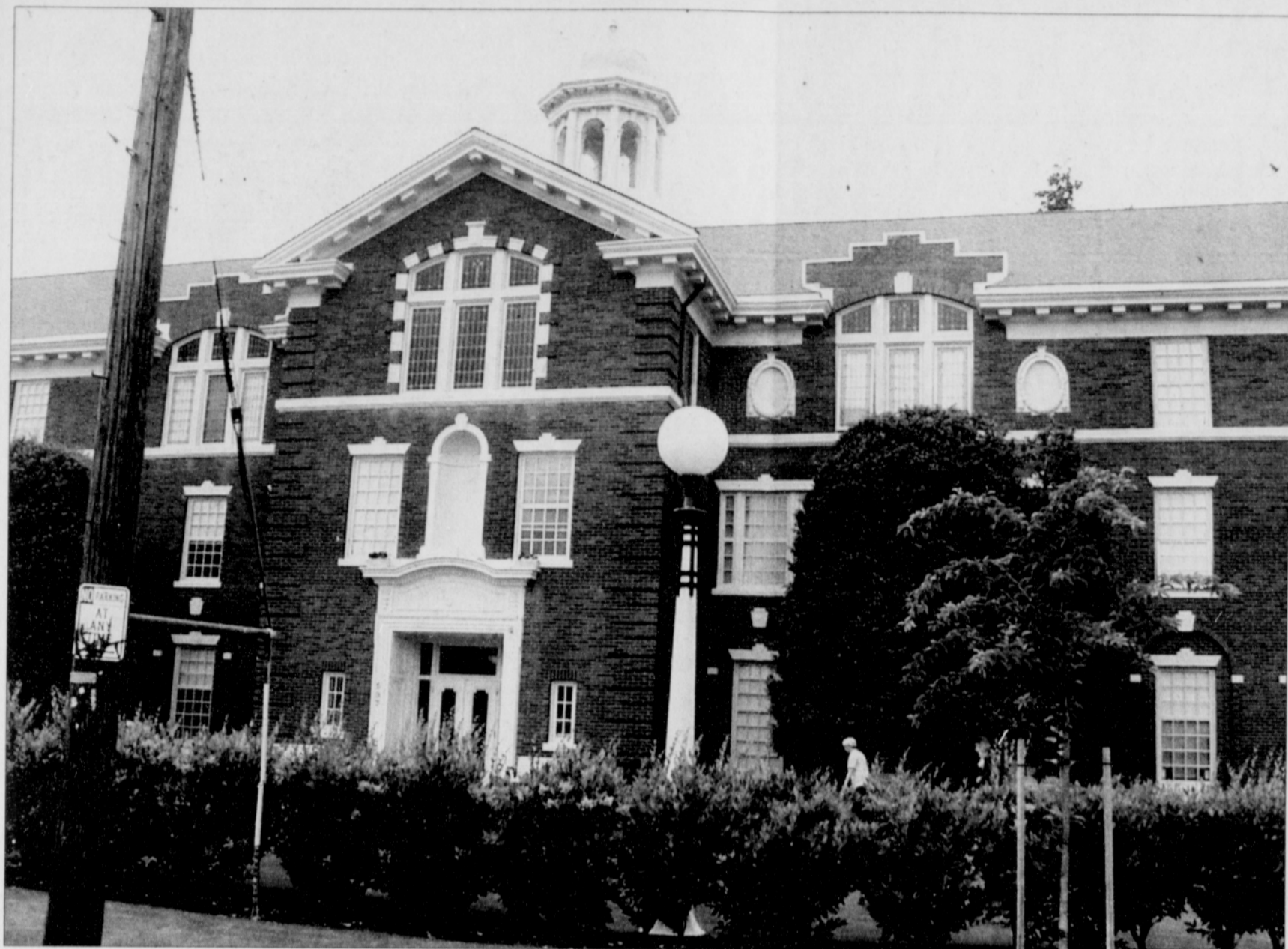
PHOTO BY RON WASHINGTON/THE PORTLAND OBSERVER The Villa St. Rose School and campus in north Portland was recently renovated into Rosemont Court, providing apartments and housing for seniors.
