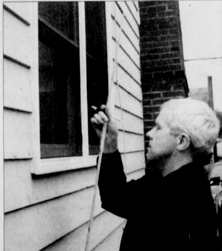
David Hall, an energy auditor for the Oregon Office of Energy's State Home Oil Weatherization Program (SHOW), measures windows on a house on Northeast 13th Avenue to find the right size of energy-efficient windows needed to weather-proof the home. PHOTO BY MARK WASHINGTON/THE PORTLAND OBSERVER
