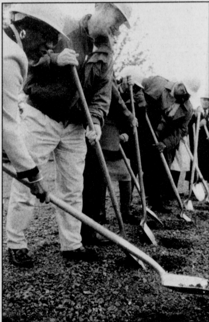
City and School officials break ground with golden shovels at the site of a new campus extension that will expand student services and increase access to adult learning programs and workforce development skills. Preexisting buildings at PCC's Cascade campus will also be updated and expanded.
