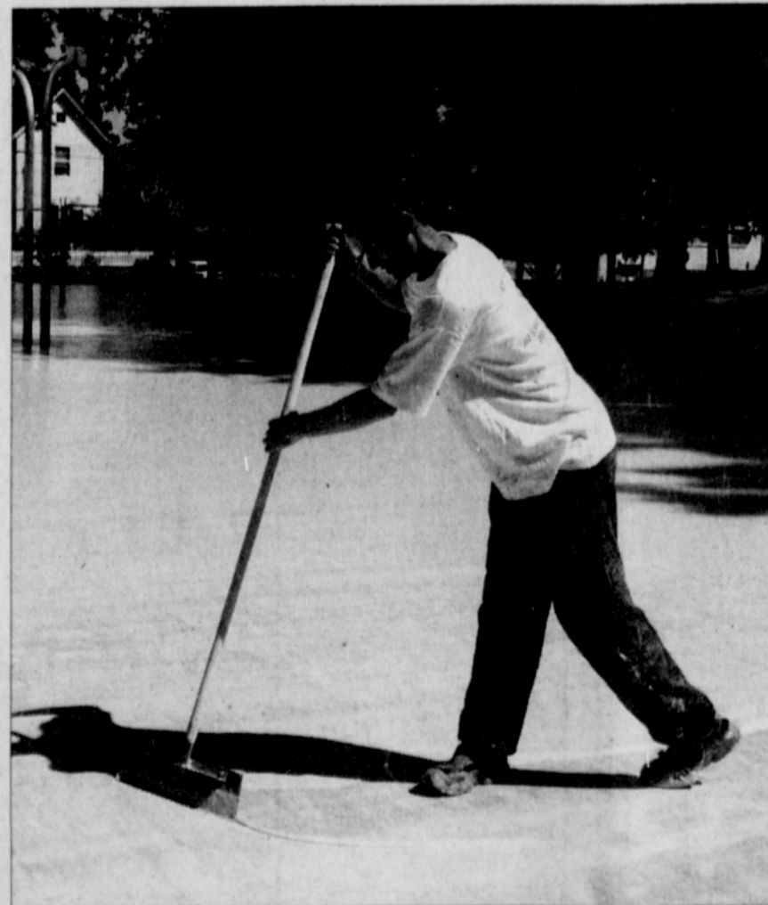
A new surface made from recycled shoes is spread Thursday across the basketball courts at Irving Park in northeast Portland. Nike is paying for the costs as part of a $2 million donation to resurface 35 basketball courts in the city. PHOTO BY MARK WASHINGTON/THE PORTLAND OBSERVER
