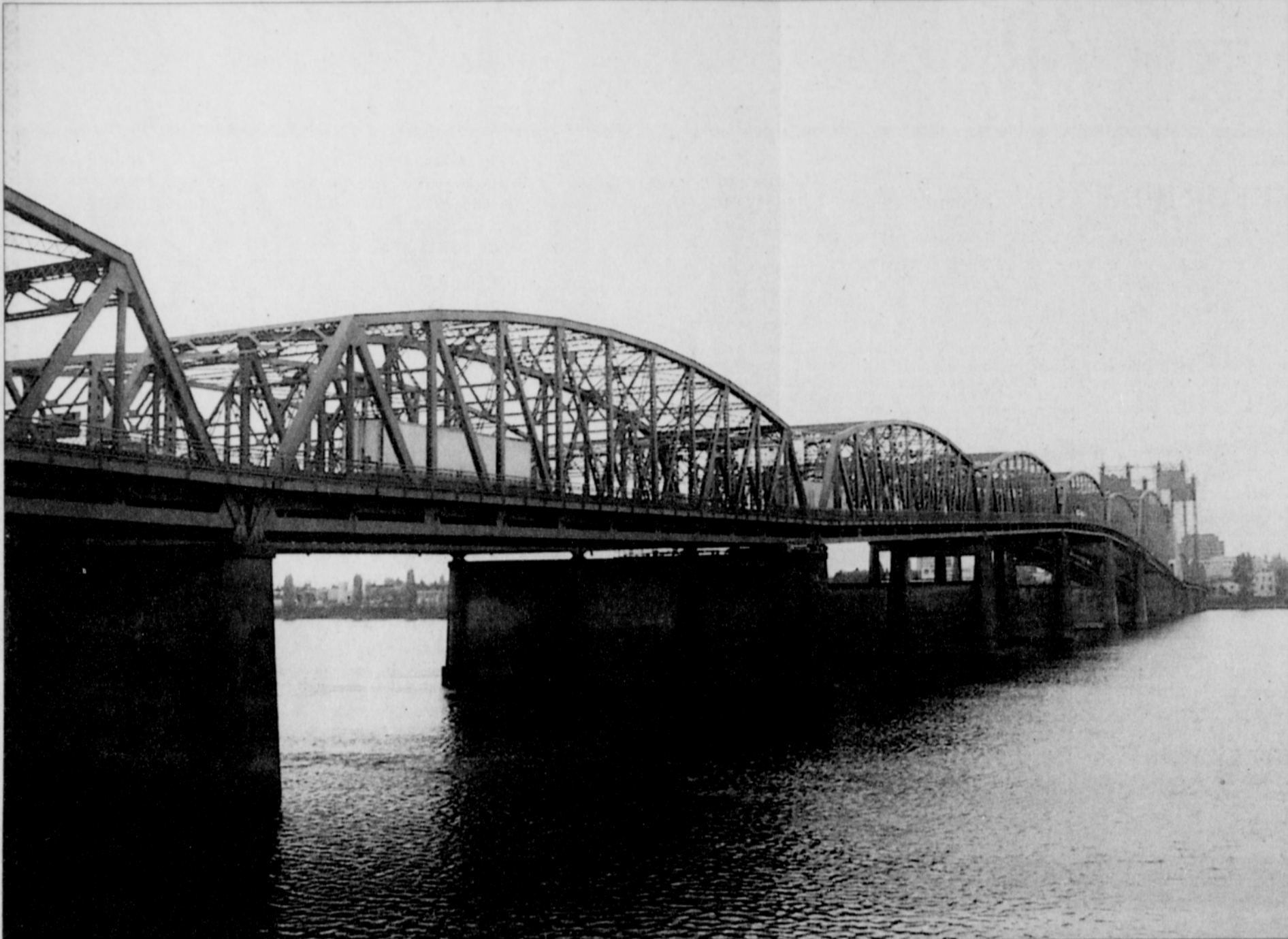
An additional or replacement span with two lanes for light rail would increase the size of the Interstate Bridge over the Columbia River from 6 to 10 lanes under a proposal by an Oregon and Washington commission. PHOTO BY MARK WASHINGTON/THE PORTLAND OBSERVER
