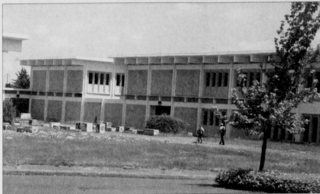
South side of former Adams high school.
