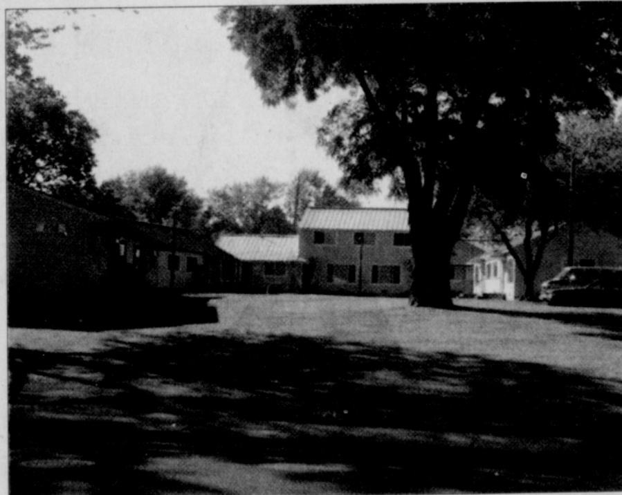
Many of the homes in Columbia Villa are World War II era structures that have been deemed obsolete.
