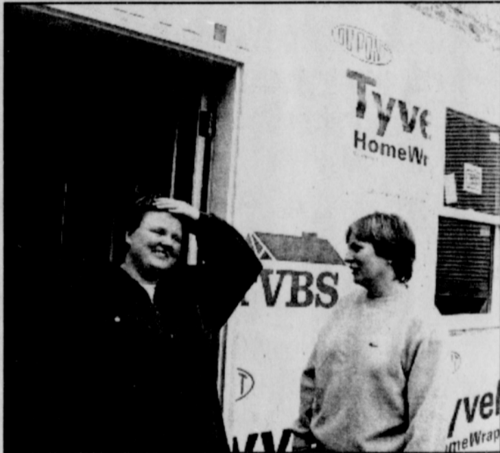
Kris Ortiz (left) and Mary Ellen Kirian of Habitat for Humanity take a breather while working on the construction of Ortiz' new home.
