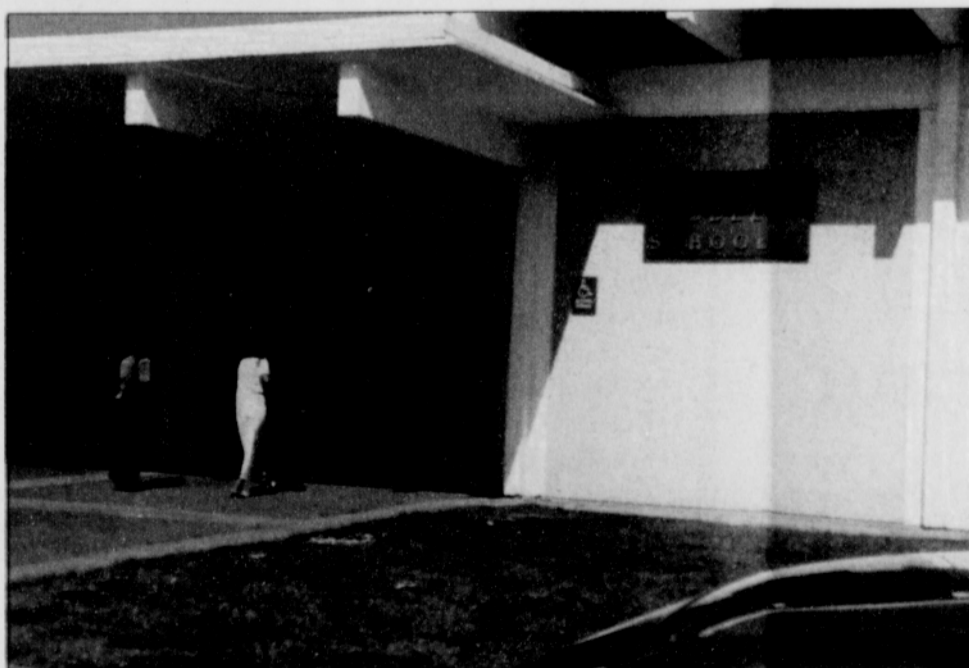
PHOTO BY MARK WASHINGTON/THE PORTLAND OBSERVER Students at Whitaker Middle School started their Memorial Day vacation two days early after tests revealed an unhealthy level of radon gas. The school took steps to circulate fresh air through the building and seal cracks in underground walls. By Monday, a new test showed a radon level of less than 1 picocurie per liter, a safe level according to the Environmental Protection Agency.
