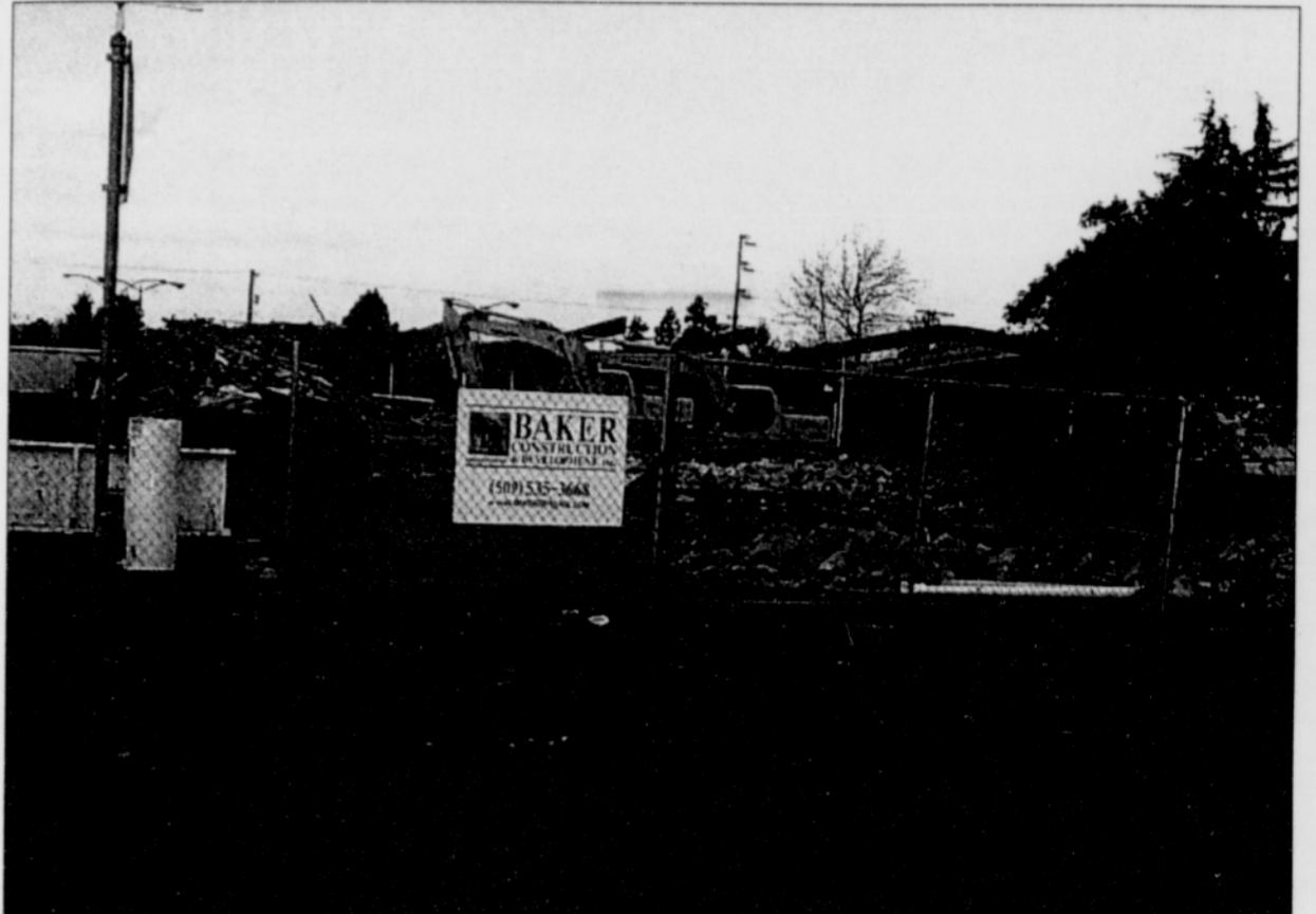
Demolition work has started at the future site of a New Seasons Grocery at Northeast 33 and Killingsworth. The market, scheduled for completion in the fall of this year, will feature natural and organic foods and also offer the best of grocery basics, creating a one-stop shopping trip for its customers.
