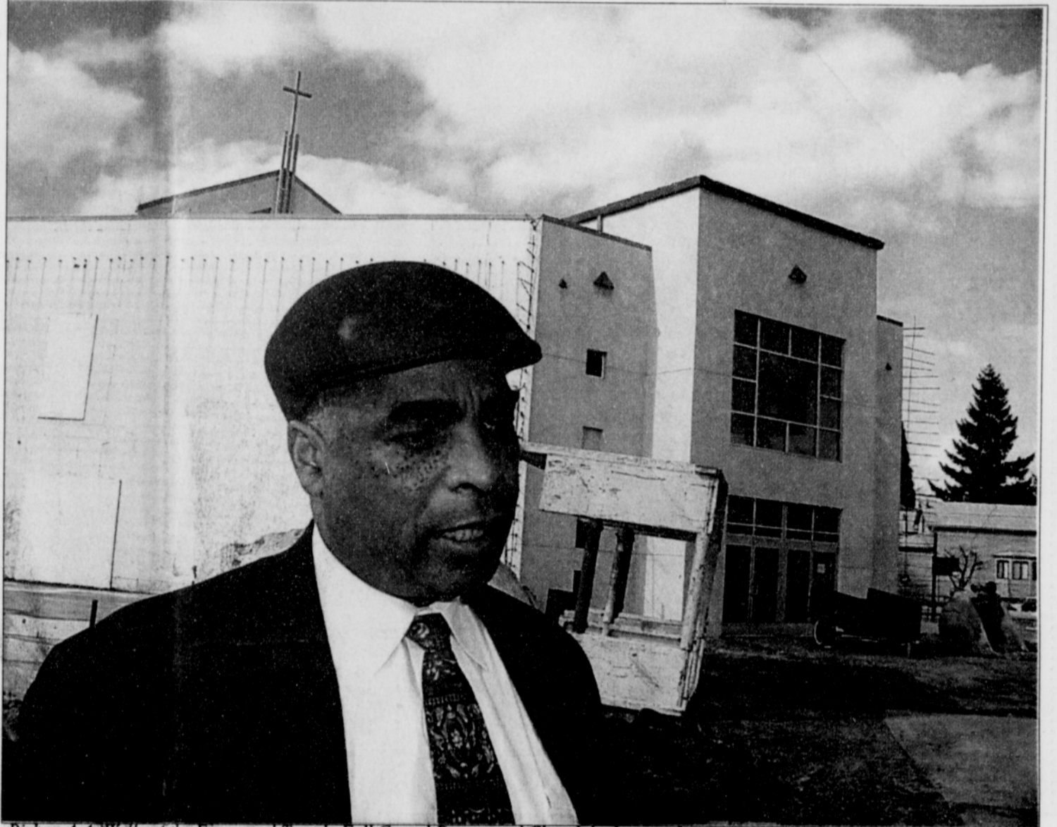
Bishop A.A. Wells of the Emmanuel Temple Full Gospel Pentecostal Church looks over the construction of a towering new church building that shadows North Sumner and Missouri along the east side of the I-5 Freeway.
