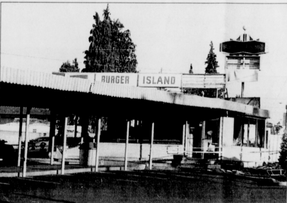
A Northeast Portland landmark is destroyed by fire.
