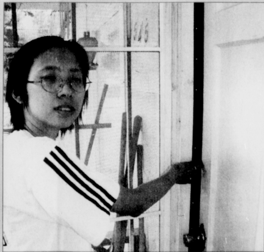
Anne Lau of the Community Energy Projects shows how insulation around the doors and windows of this Southeast Portland home will add comfort and lower heating bills this winter. (Photo by Michael Leighton/Portland Observer)
