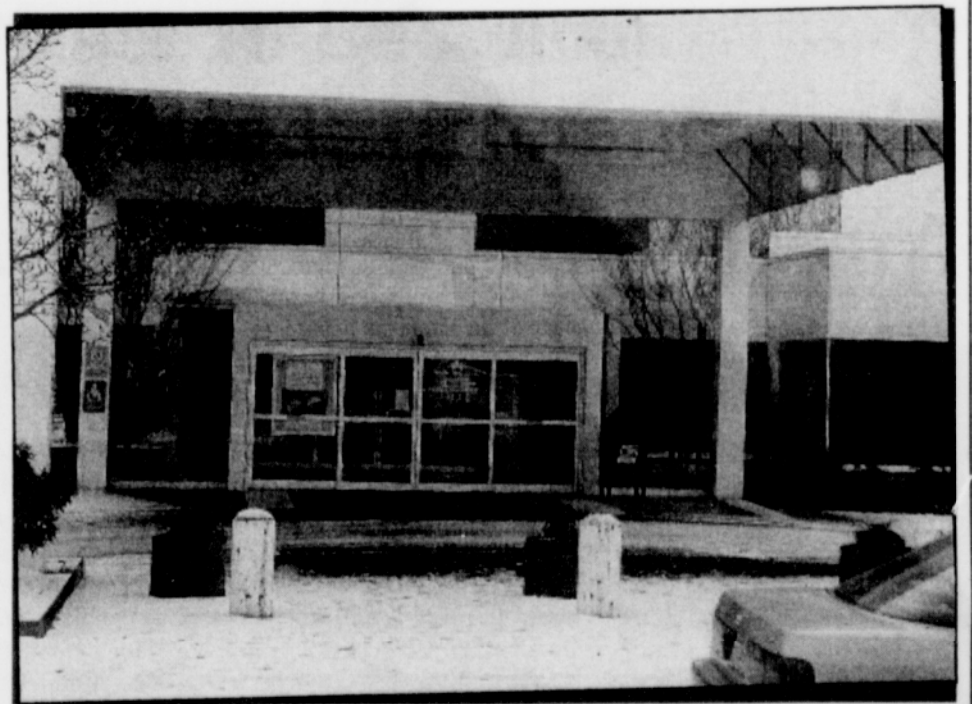
Former Bess Kaiser
