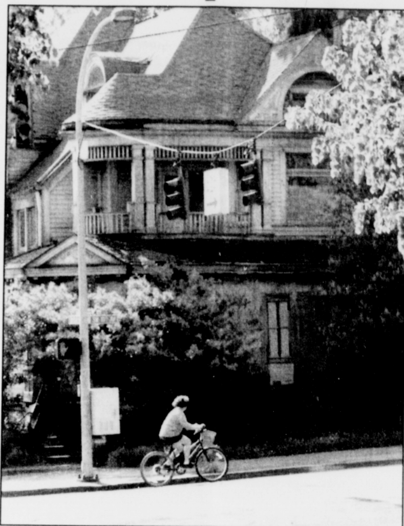
The Simon Benson House, a downtown Portland historic landmark that was built in 1900, has been closed for several years but will get new life after it's moved to the Portland State University campus by this fall. It is expected to reopen eventually as a new home for the PSU Alumni Association and PSU Office of Alumni Relations. (PSU photo by Brian White)
